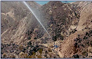
Construction Pre-Wet / Sprinklers
