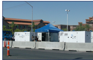
Sewer Bypassing with Qualified Personnel
