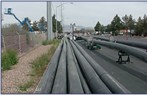
High Density Polyethylene Fusing "HDPE Fusing"
